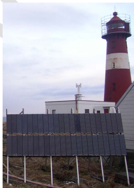
Figure 2 Grasøyan lighthouse solar array
